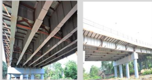
Road over bridge at Behrampore, Kishangarh
