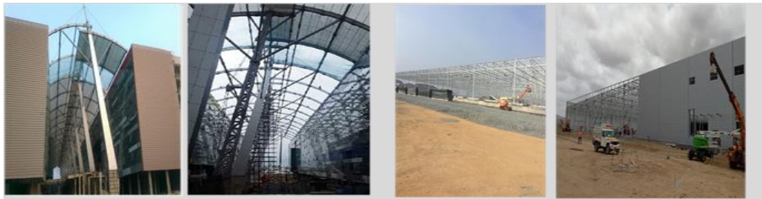
Canopy Structure at TCS Hyderabad
