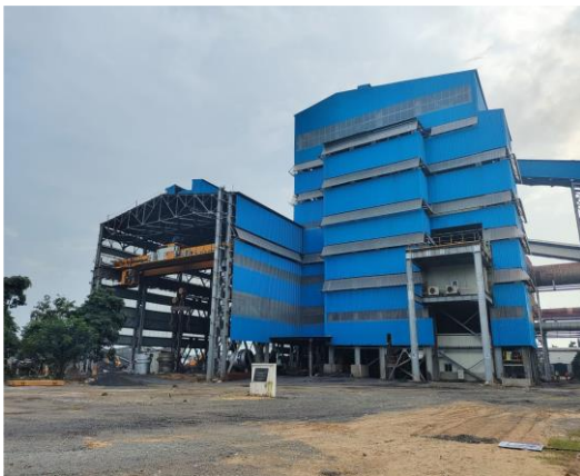
FURNACE BUILDING AND CAST BAY
